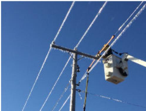
High winds and ice can affect power lines in a way that makes them gallop. Strong winter winds can cause ice to build up on one side of a power line. When this disproportionate buildup occurs, it changes the flow of air around the line, which can then cause it to start bouncing, potentially damaging the lines, causing power outages and even making the lines fall to the ground.
